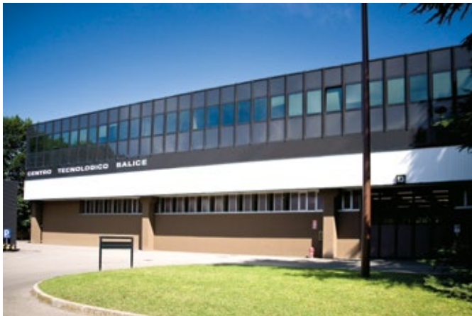
Salice Technological Centre in the Novedrate factory
