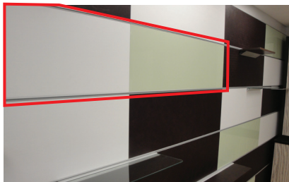
Snap in panels installed
